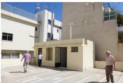
Roof top, Terrace with service rooms
