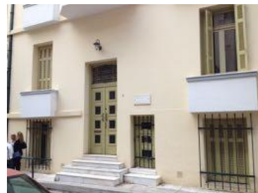
Oriniou 3, Main Entrance between Ground and First Floors
