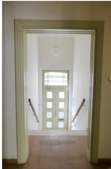
Main Entrance and staircase from street
