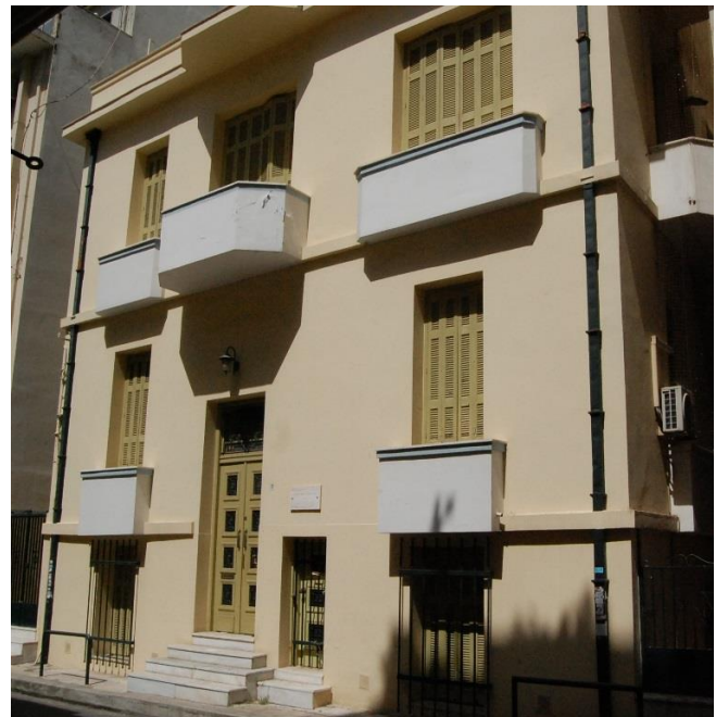
The New Home of the Canadian Institute in Greece
