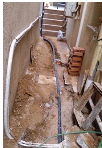
New drainage pipes in trench
