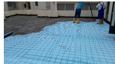
Thermal insulation layer covered by concrete
