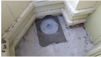
Improved balcony drain
