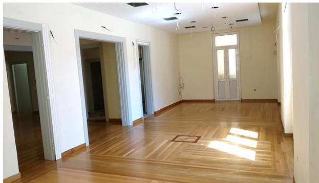
Lecture Auditorium nearing completion
